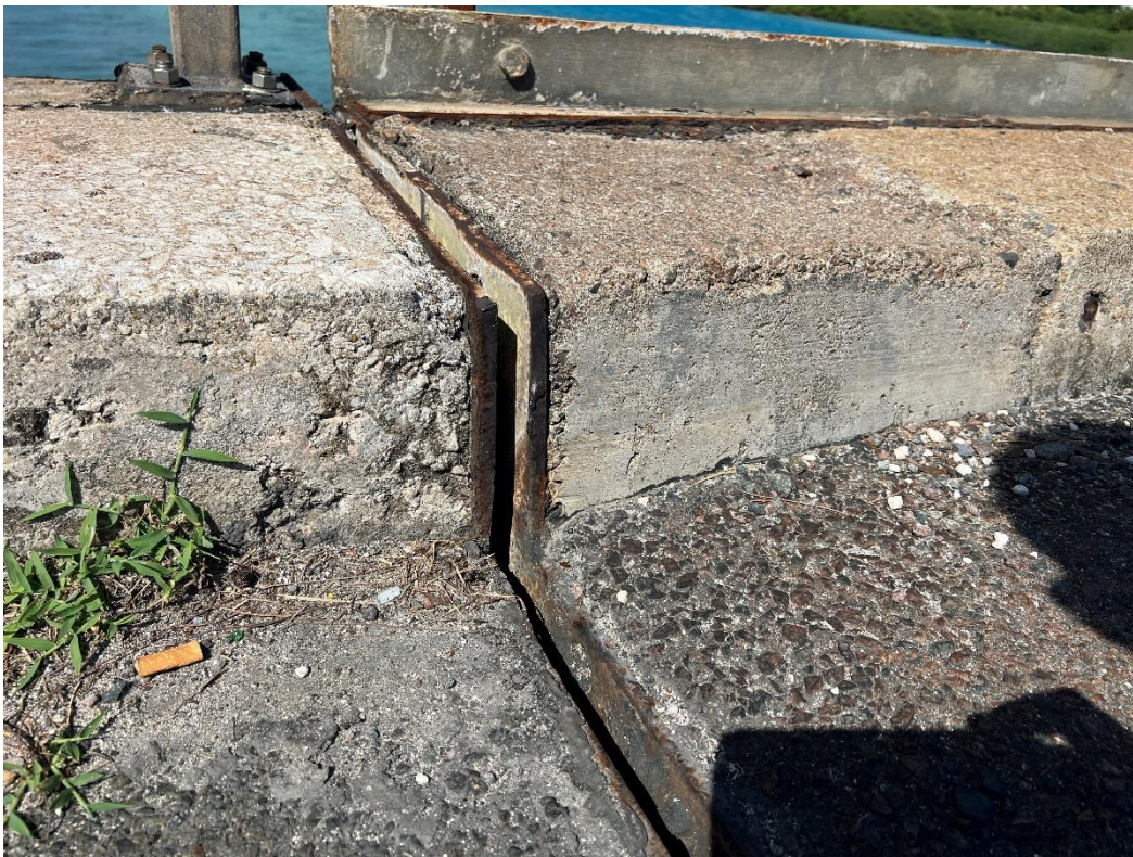
Photograph 2 – End plate at curb location
