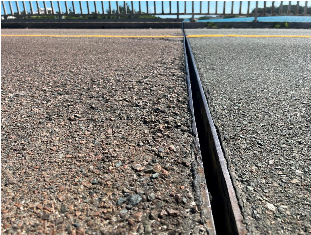
Photograph 1 – Existing end plates
