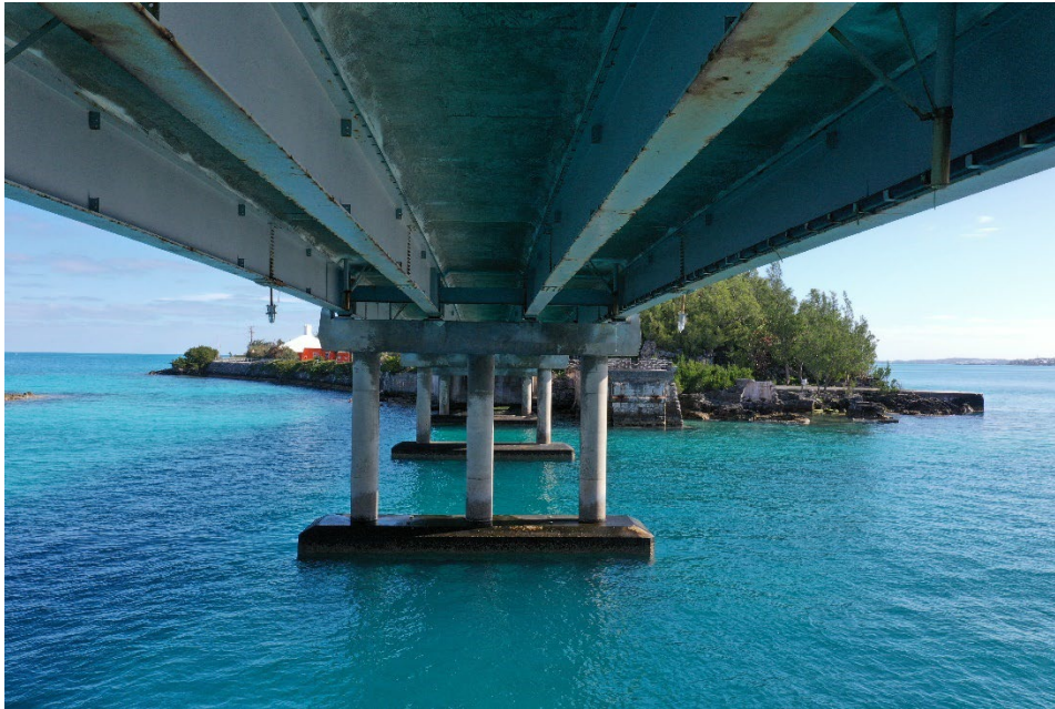
Photograph 13 – Span 4 Main Girders.
