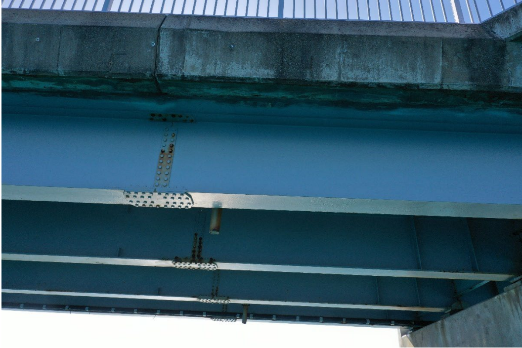
Photograph 5 – Span 2 plate girder splice connection.
