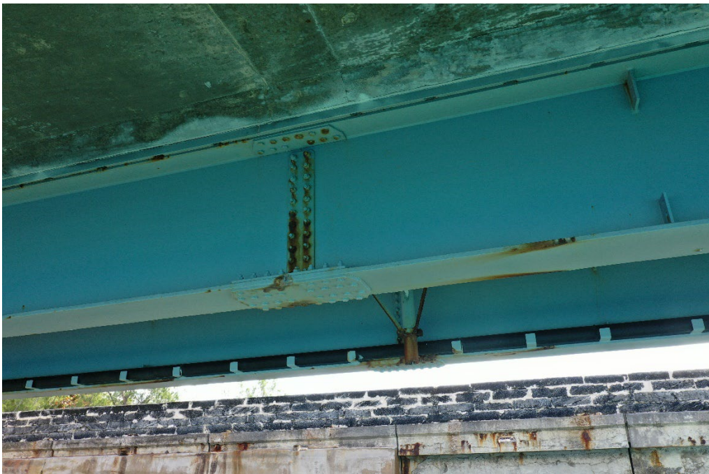
Photograph 18 – Span 7 Main girders and splice connections(1).
