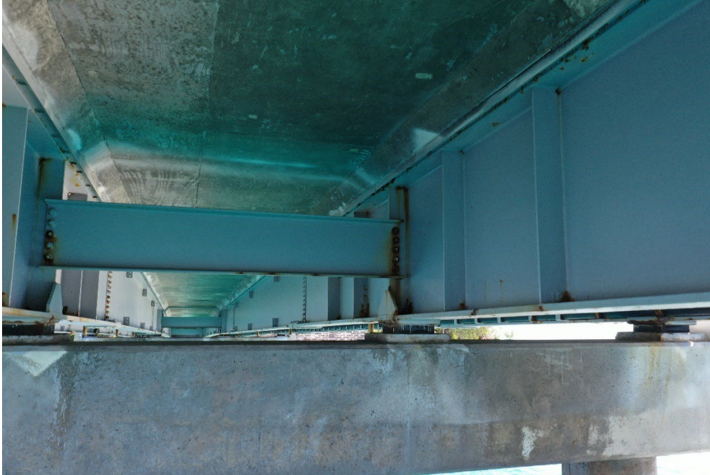
Photograph 15 – Span 5 Main girders.
