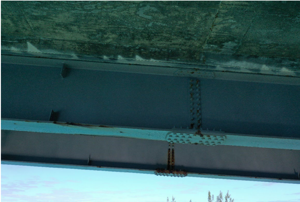
Photograph 17 – Span 7 Main girders and splice connections.
