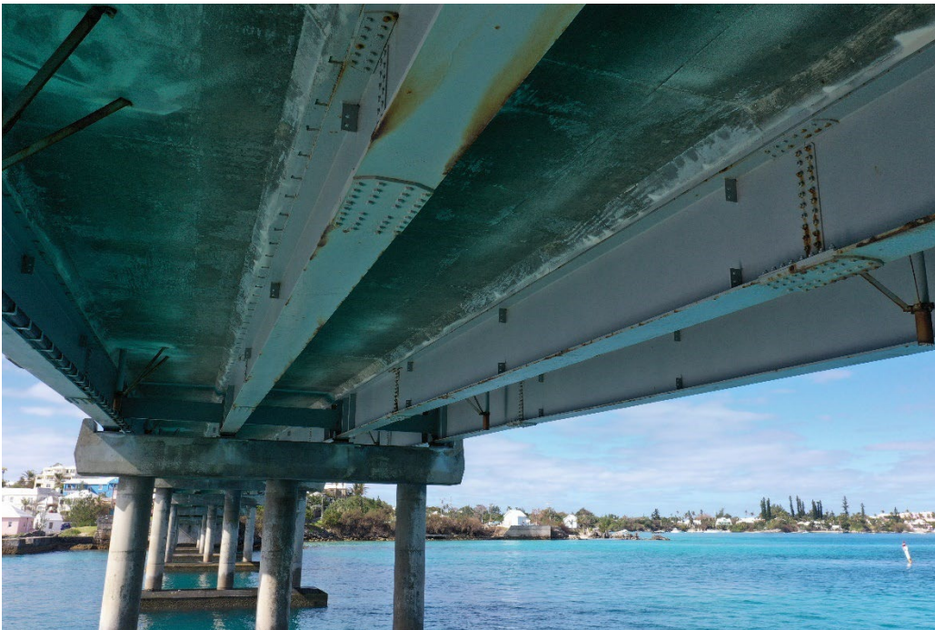
Photograph 16 – Span 6 Main girders and splice connections.
