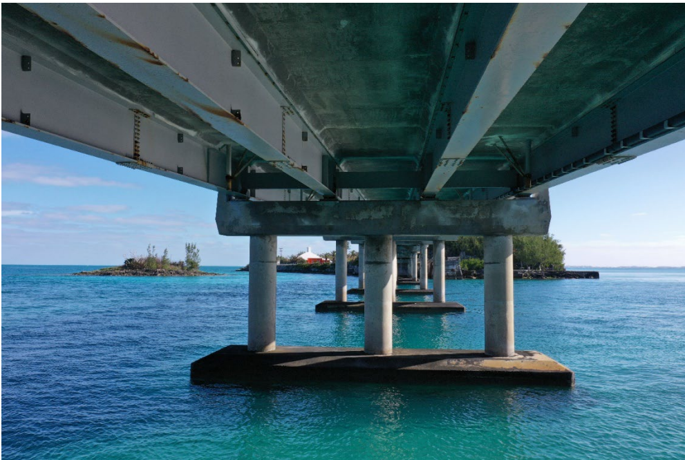
Photograph 2 – Span 1 main girders.
