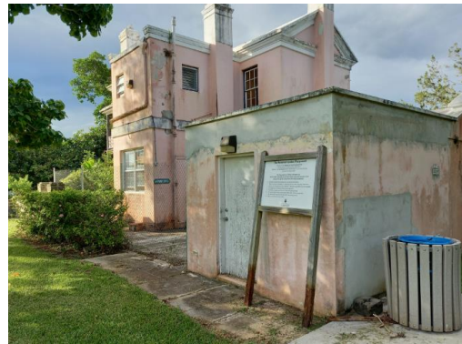
BGL- 34: Northeast Elevation
