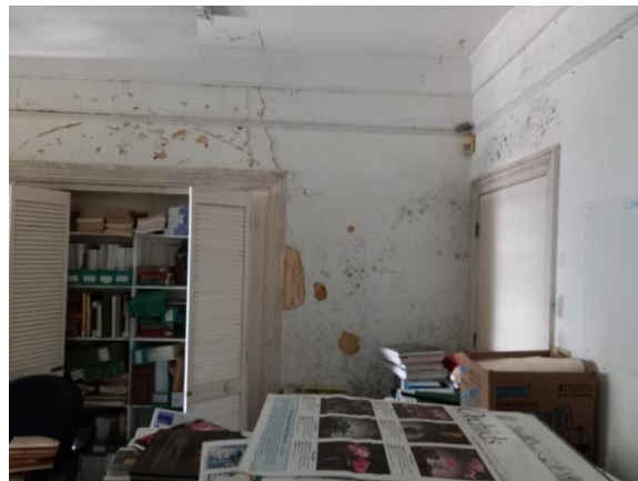
BGL- 32: Room 105, D5, D6 & S8
