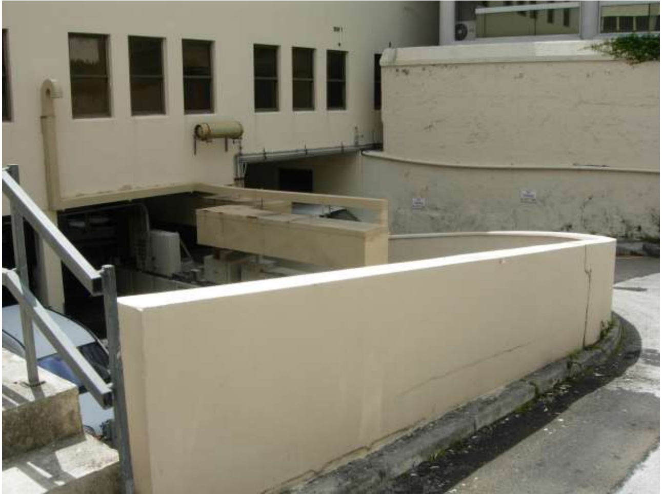
West Elevation (Car Park Access Wall and Boundary Wall)
