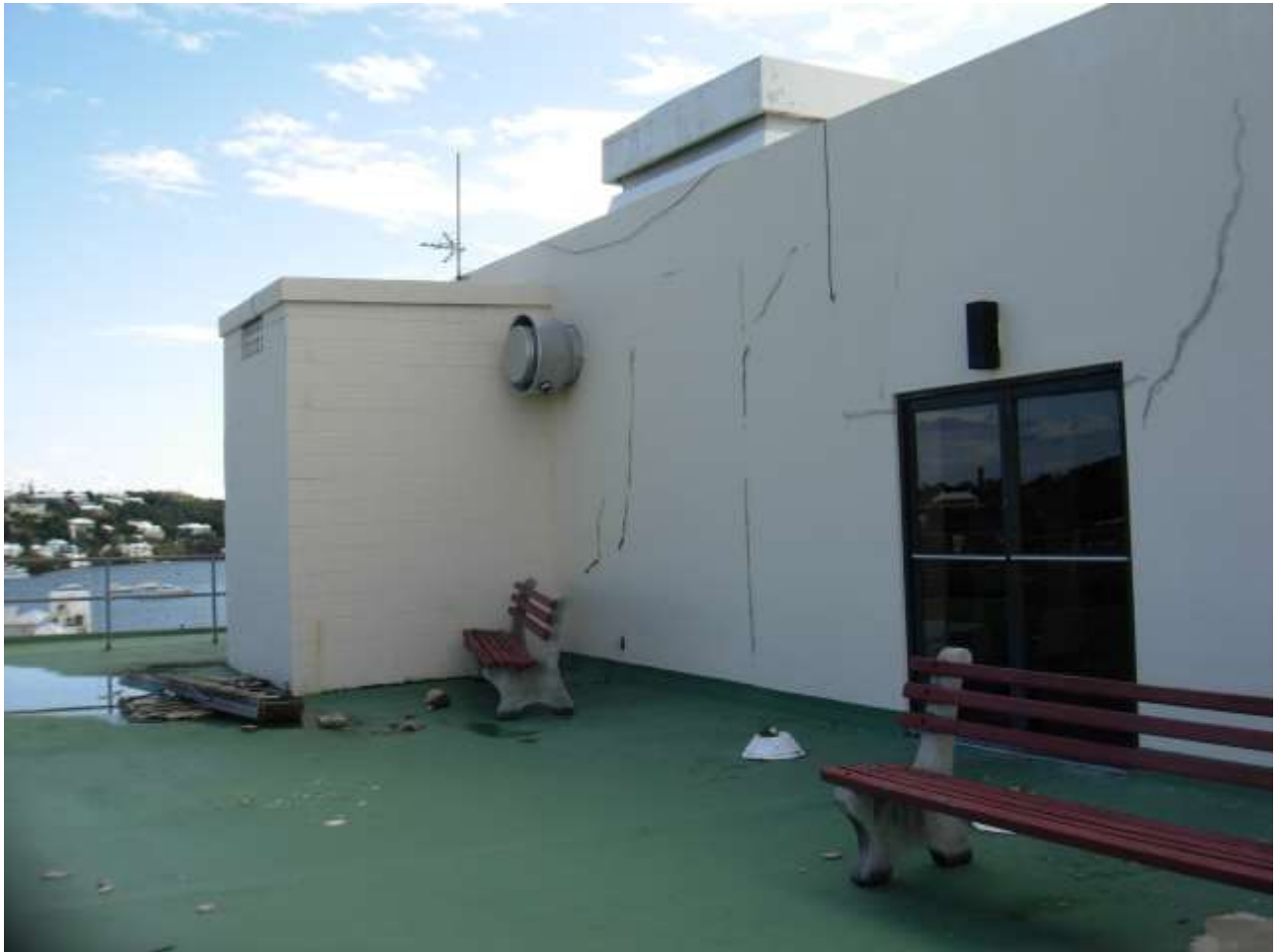
4 th Floor Sun Deck
